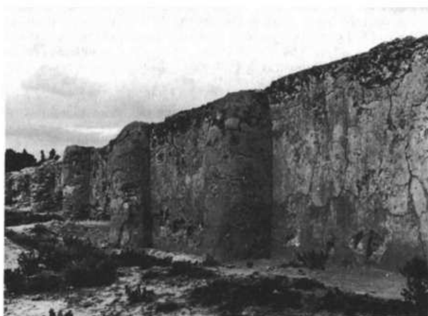
PLATE 10.5 The great lake of Ruḳḳāda, near Ḳayrawān. Massive embankments served as a breakwater against waves whipped up by the wind
